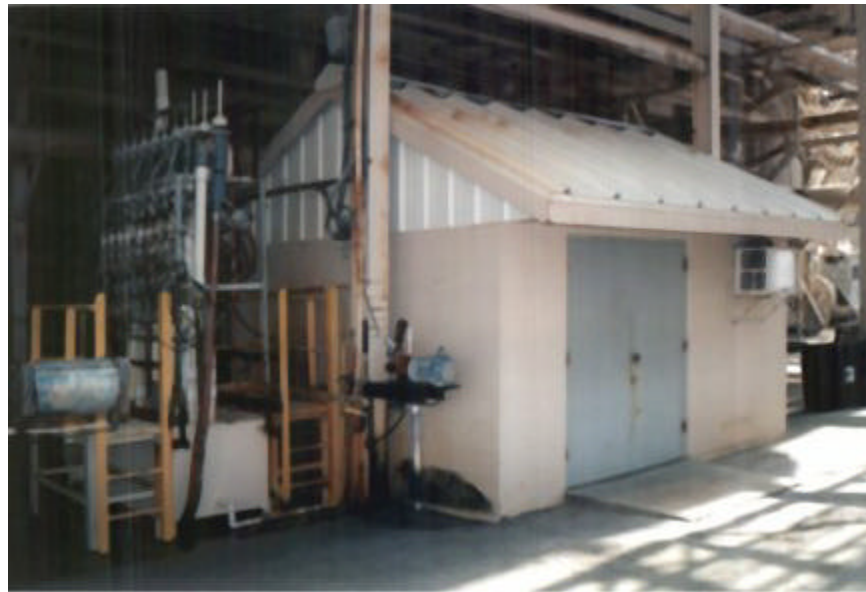
FIGURE 6. Analyzer Building with Sample Presentation for Eight Sample Streams
